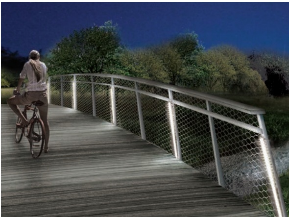
Led lighting on railing
